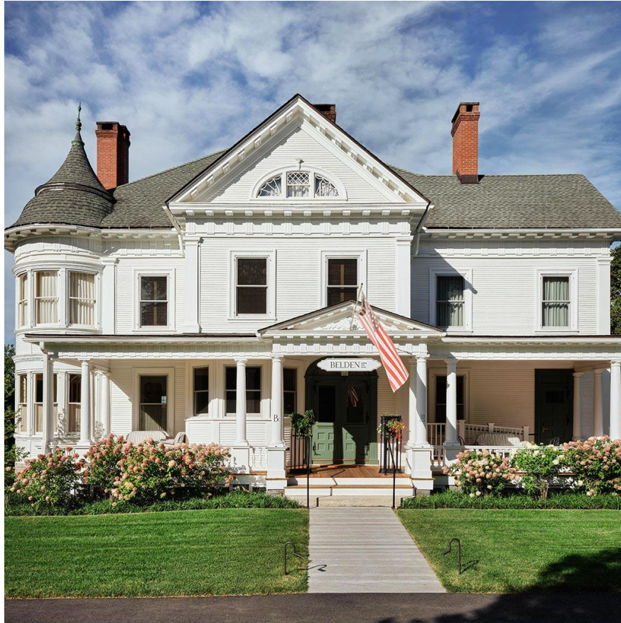
Belden House & Mews breathes new life into an 1888 Victorian home. © Belden House & Mews
